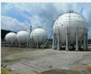
Natrium Processing Facility Caiman Energy Designed and built by CB&I Inc.
